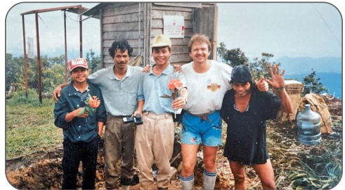
Building a transmission tower, 1990
